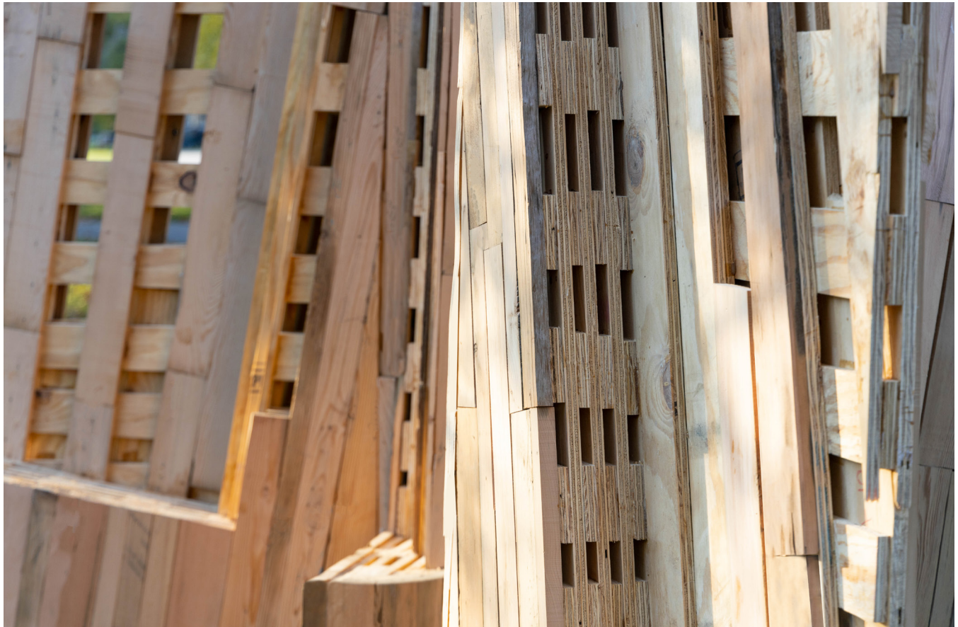
Figure 3. HoloWall showcasing the thickening and thinning of layers and varied porosity.
