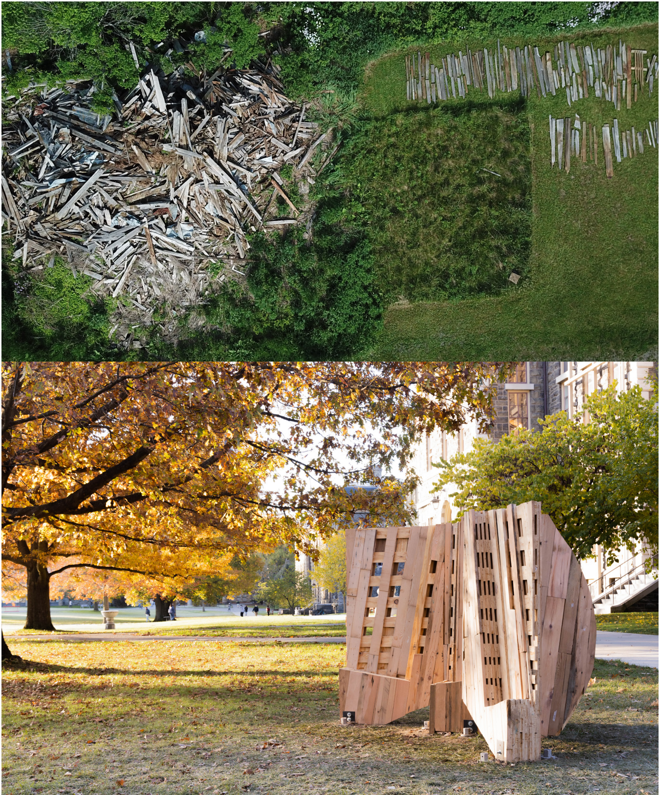
Figure 1. Waste wood from a local collapsed barn that were used for the project (Top) and HoloWall installed on site (Bottom).
